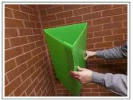
Step 5: Insert zip ties into the top and bottom of the tab panel. Secure ties.
